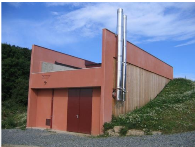
Chaufferie collective – Izeron – 38
